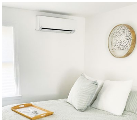
Ductless ASHP indoor wall unit
