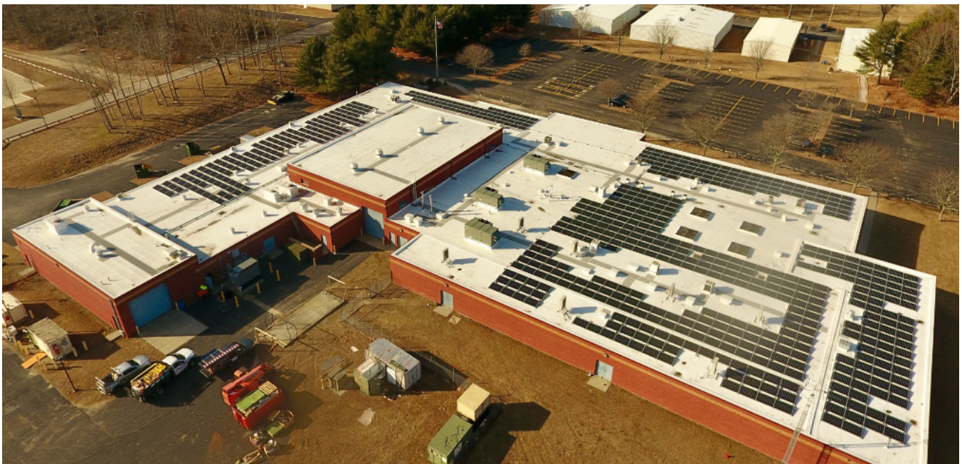
The National Guard installed the largest roof-top solar system on state facilities, with a 210 kW nameplate capacity.
