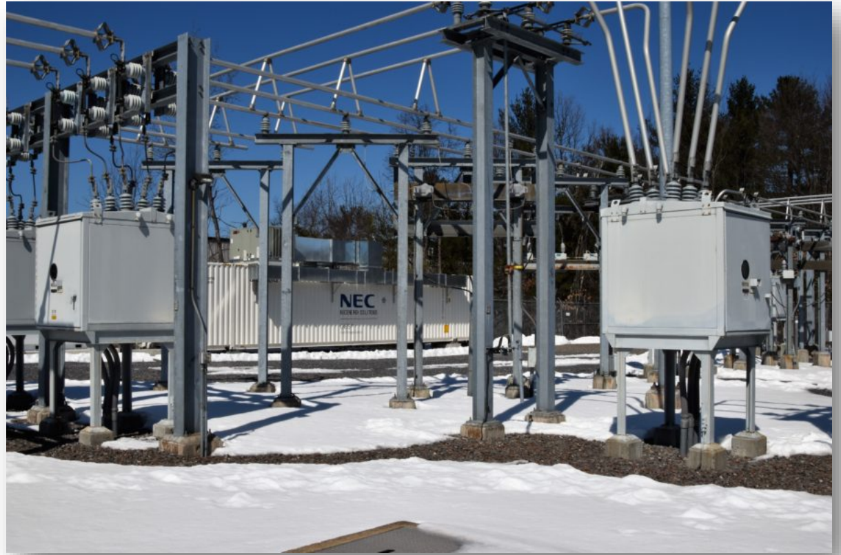
Photo by Clean Energy Group, March 2017.
