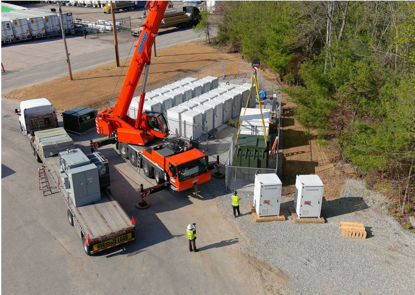
Installation of a 3MW/9MWh grid-scale battery storage system
