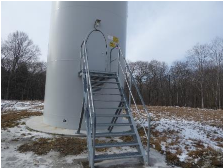
Figure 18. Wind Energy System Tower Base
